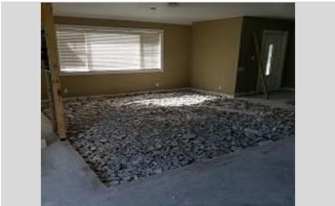
Filed Lower Living Room with old Tiles, Cement will cover Now
