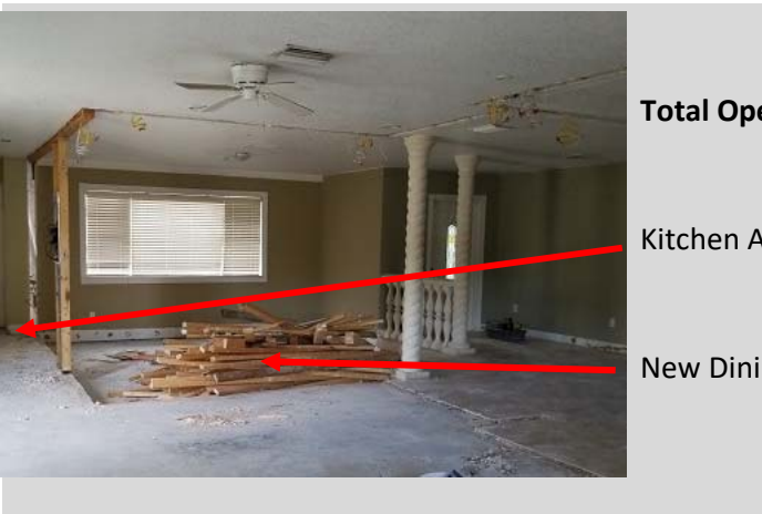
Filed Lower Living Room with old Tiles, Cement will cover Now
