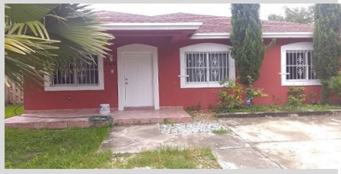
(BEFORE) Original Condition
